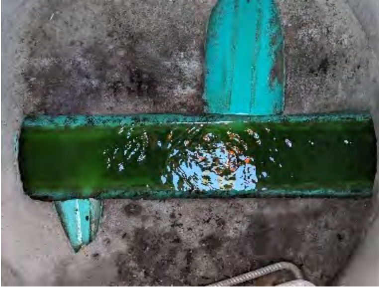
12. CB-4 and CB-5 on Campbell connect to COMB-C (green dye)
