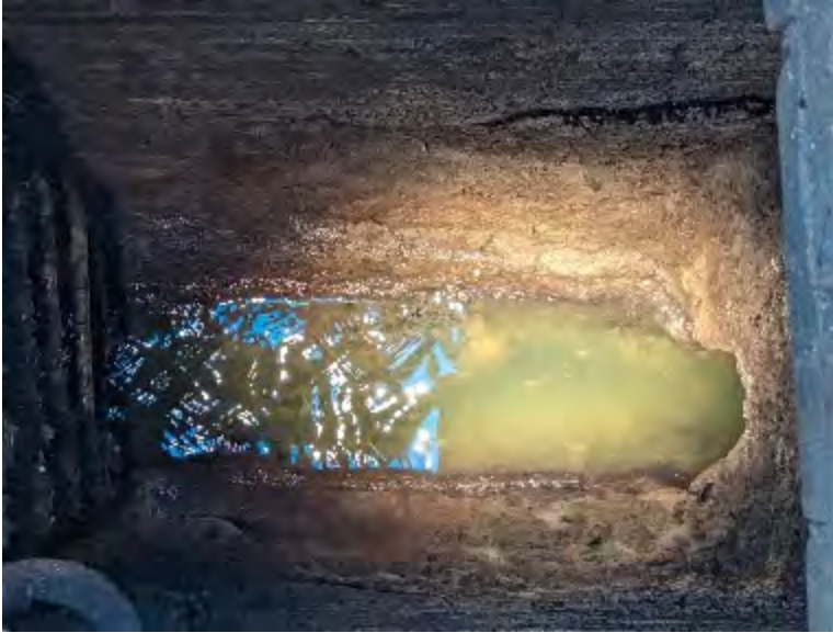
4. CB-1 and CB-2 on Randolph connect to COMB-A (Green dye)
