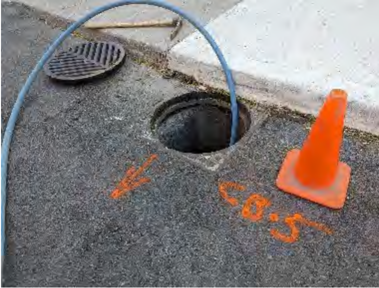
10. CB-4 and CB-5 on Campbell connect to COMB-C (green dye)
