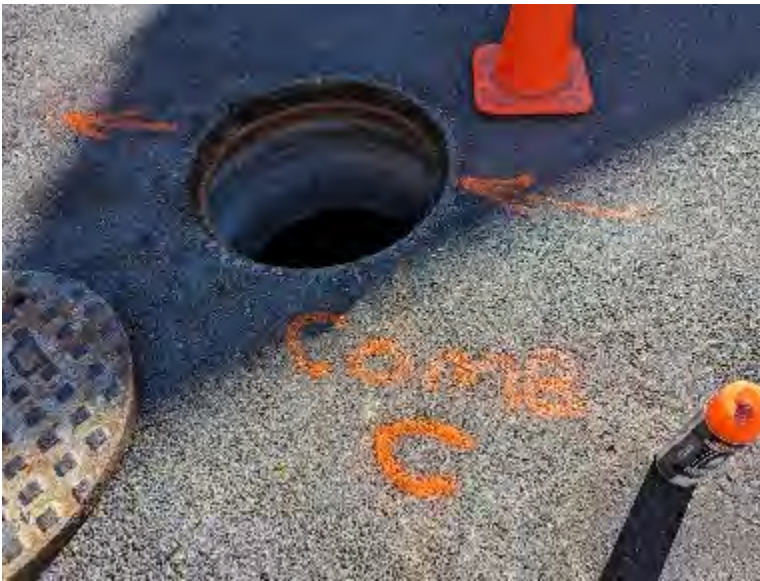
11. CB-4 and CB-5 on Campbell connect to COMB-C (green dye)
