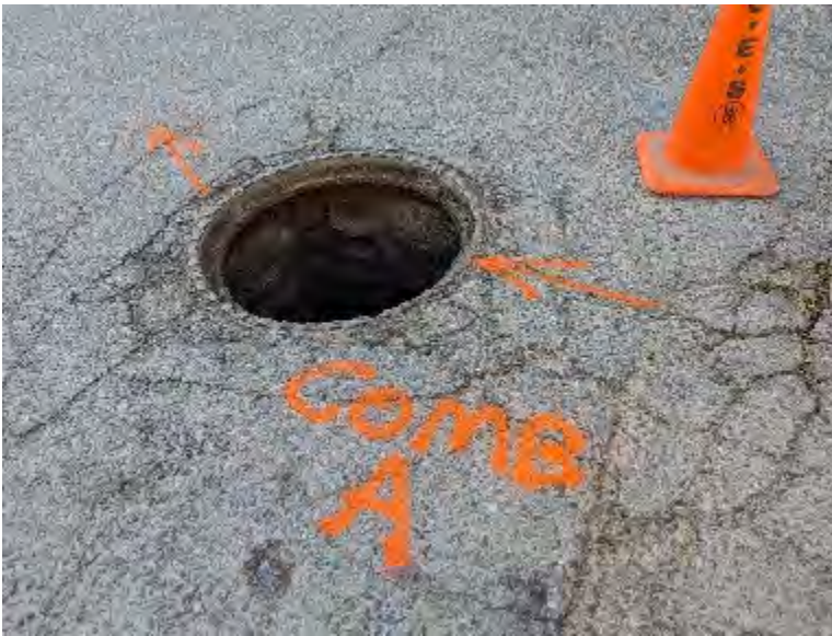
3. CB-1 and CB-2 on Randolph connect to COMB-A (Green dye)
