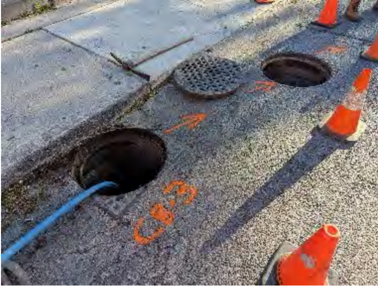
6. CB-3 Ernest connect to COMB-B (green dye)
