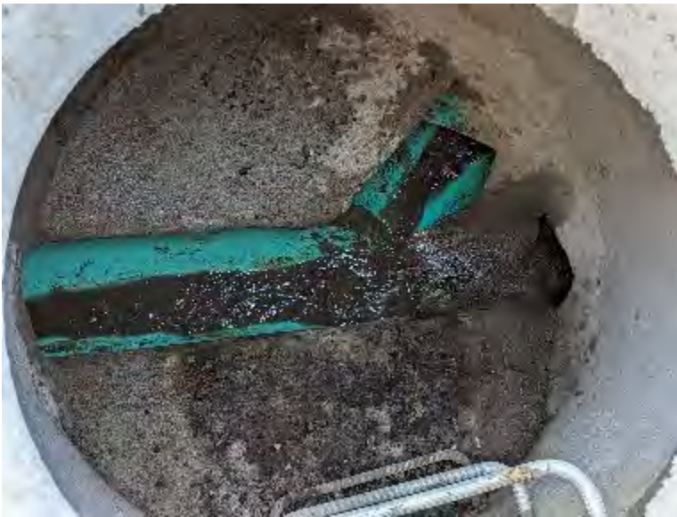
15. CB-7 on Campbell connects to COMB-D (green dye)
