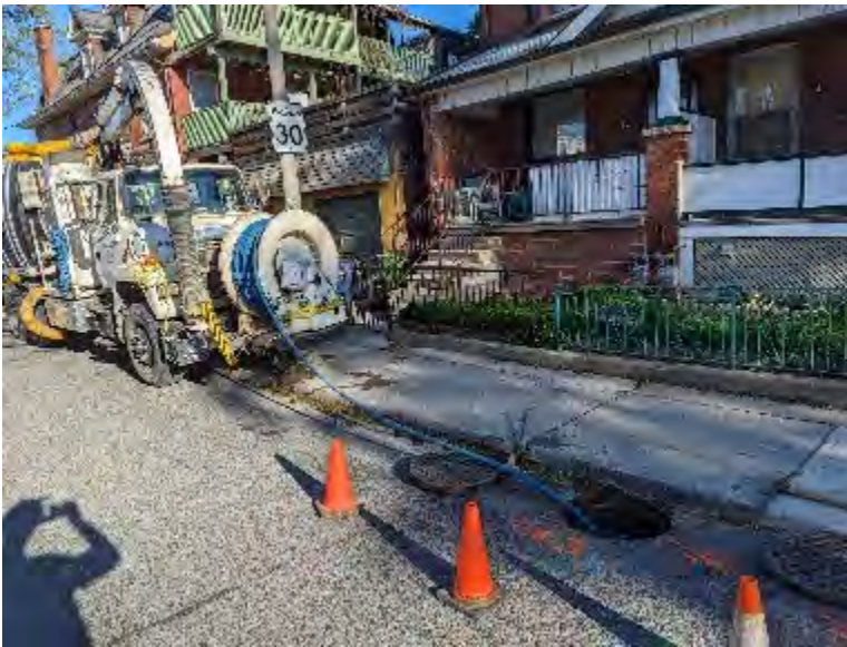
5. CB-3 Ernest connect to COMB-B (green dye)
